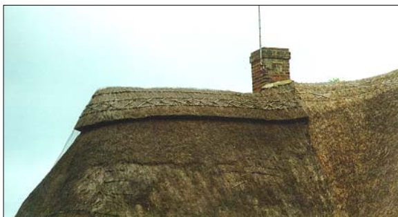
Photograph 6 - A block cut ridge
