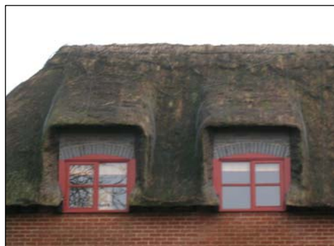
Photographs 12 and 13. Narrow valleys, higher thatch draining onto lower thatch, anomalous vertical thatch panels over and on the cheeks of tall eye brow windows.
