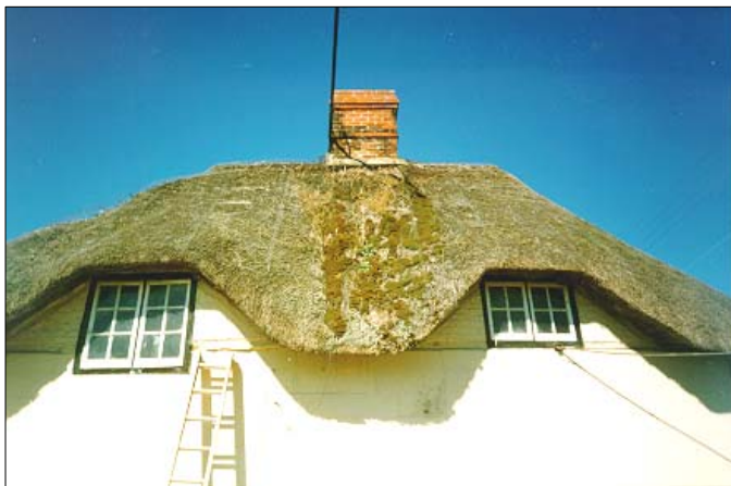
Photograph 1 – Time for action. Note the concave dip and fixing spars visible on the left hand hip, the stranded flashing around the chimney, and the heavy build up of moss indicating permanently damp areas.
