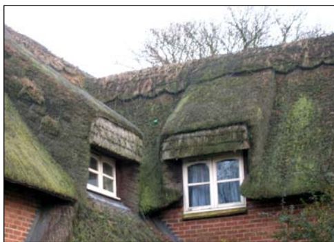
Photographs 12 and 13. Narrow valleys, higher thatch draining onto lower thatch, anomalous vertical thatch panels over and on the cheeks of tall eye brow windows.
