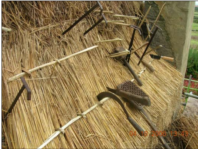
Photo 4 - Close up of combed wheat being laid. The provision of a horizontal bond formed of hazel liggers (which will eventually be concealed – see Diagram 1) highlights a major difference to laying in the Long Straw style. It should be noted however that the bond in most historic buildings within the District is formed by tying a small portion of each bundle to its neighbour – a straw bond.
