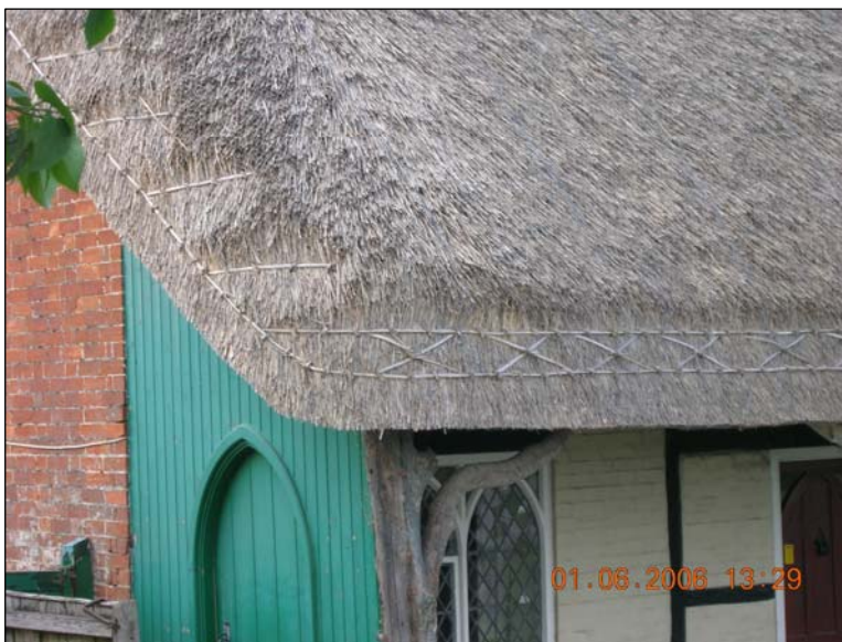
Photograph 3 - Close up of long straw thatch – note distinctive straps fixed at the eaves
