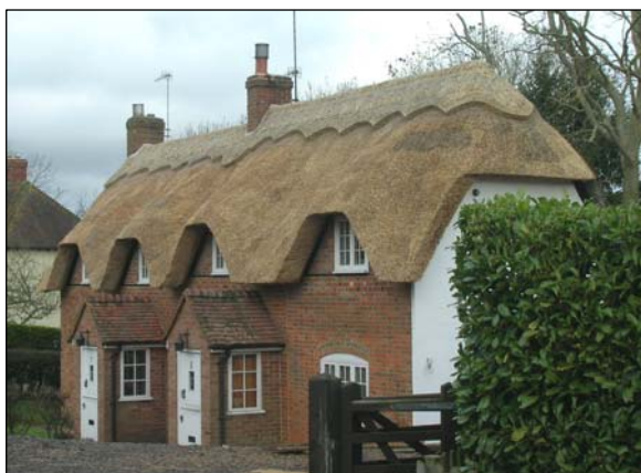
Photograph 7 - decorative block ridge
