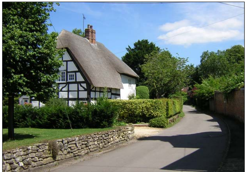
Photo 5 - a roof with a weathering coat of combed wheat – note the crisper lines and denser appearance of the thatch
